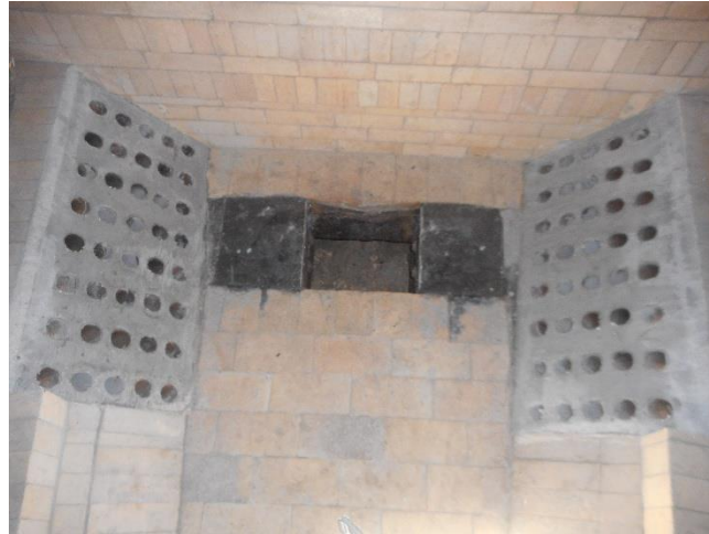
Direct “orange-juice” ventilators on each side with the damper inlet in the center
