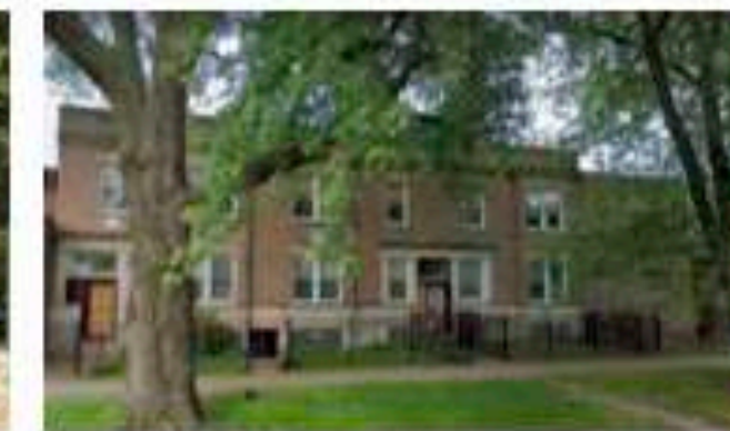
Vacant buildings provide a base for storage and processing
